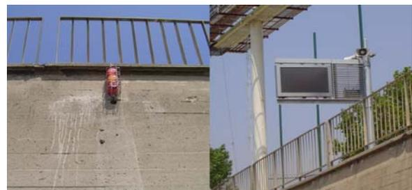
Figure 2: Optical-acoustical signal, information panel and loudspeaker system.
